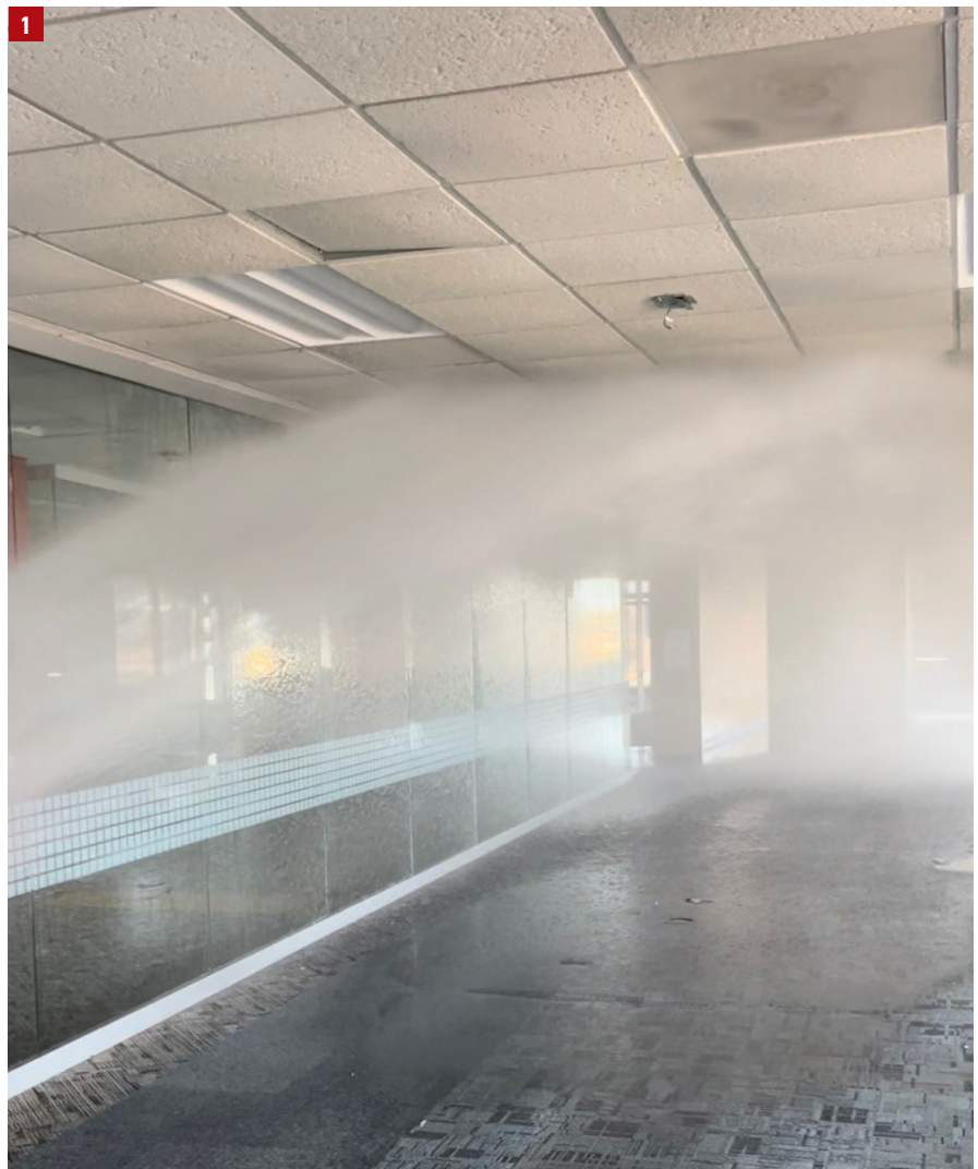
1. The BLADE™ stream nozzle in use at a commercial structure. (Photos courtesy of HEN.)
